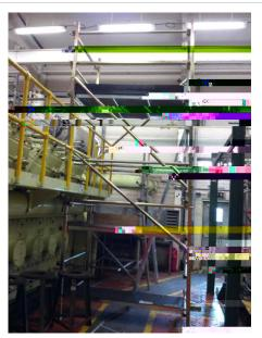
Figure 2: Tower 2: 2.4  $\times$  1.4  $\times$  4 m, 2 Standards offset on gantry of Compressor K40.
